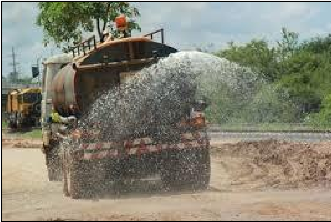
Water Sprinkling at Site
